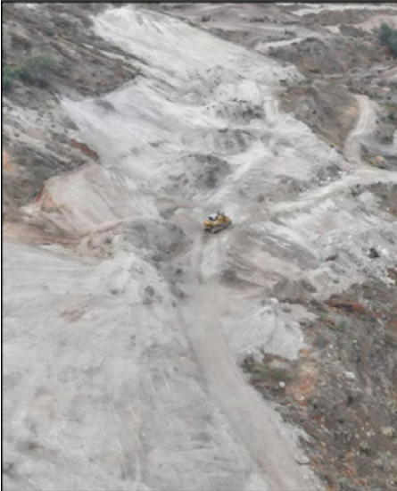
Figure 3. Earthworks at the Merrill-Crowe Plant and Pregnant Pond Areas
