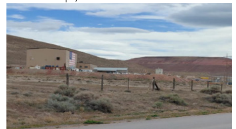
This is but a part (with the main Admin and processing buildings) of the sprawling Florida Canyon Mine, now undergoing Modernization and Expansion thanks to Record Gold Prices!
