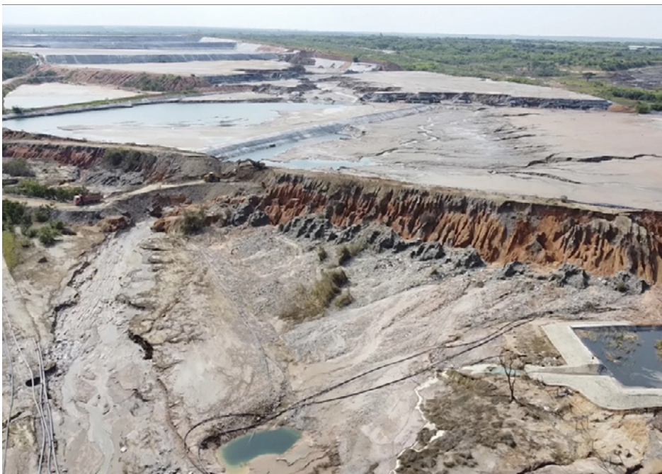
The tailing dam failure at Sino-Metals Leach Zambia. Source: AP News
