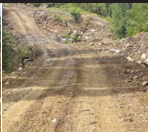
Upgrade of all-season access road for its flagship Kenbridge Nickel project in Ontario.
