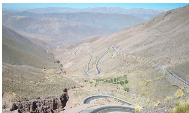
Highway to our drill site in Jujuy Province
