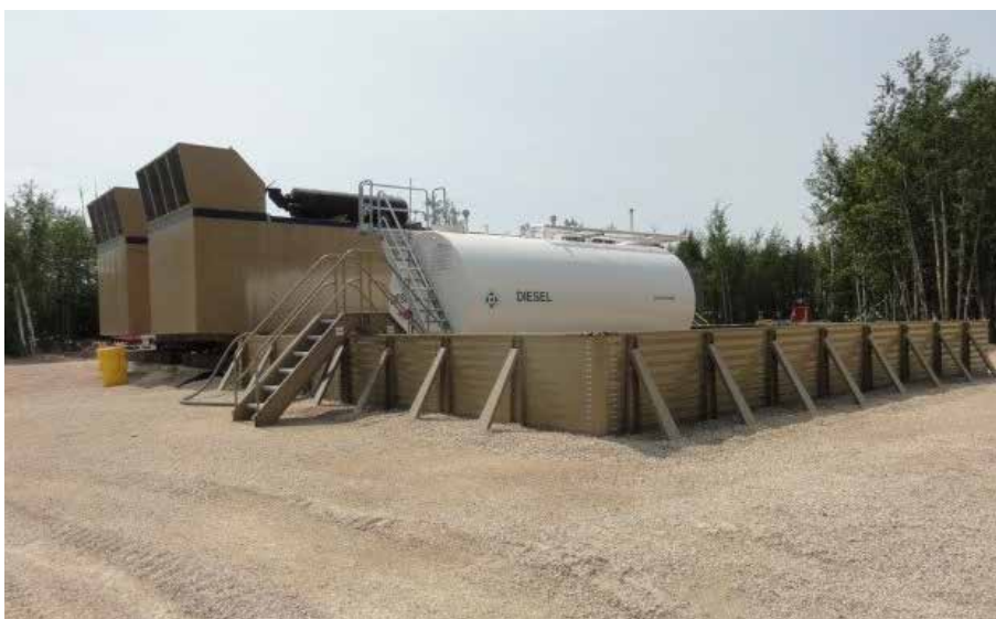
Completed diesel generators with fuel storage and containment
