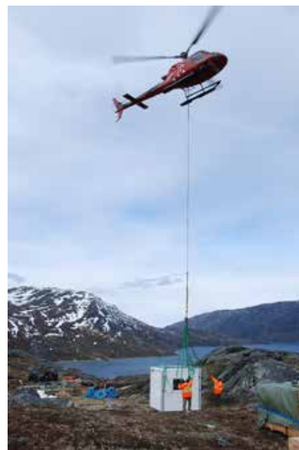
Helicopter slinging a portable refuge shelter into place
