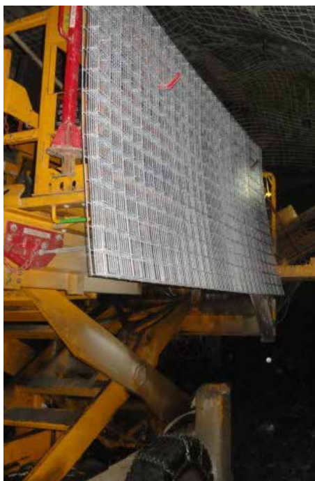
Maclean bolter screening and bolting the main ramp
